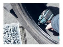
10. Then screw two 40mm low profile head screws to into each side piece. You can do this carefully by eye or measure and mark with chalk first.
