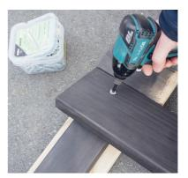
7. When the end cross pieces are in place the inner cross pieces can be positioned and screwed on.
